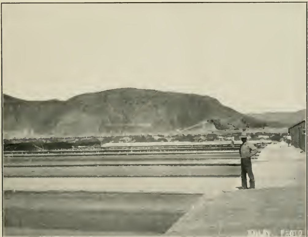
BORIC ACID CRYSTALLIZING VATS—HUMPHRIES'S WORKS, DAGGETT, SAN BERNARDINO COUNTY.
